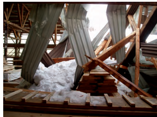
Figure 4: Snow pressure caused the collapse of a hall roof, Waldstatt 2006. (Source: Thomas Egli)
